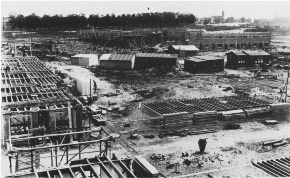
21. Olbertz dwellings under construction, circa 1923
